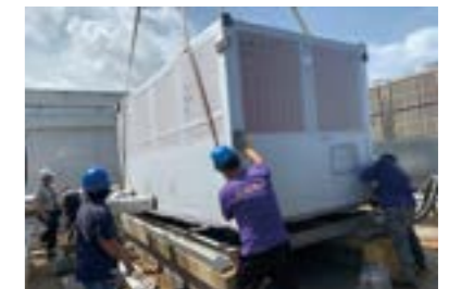
Renewal of air conditioning heat source equipment
