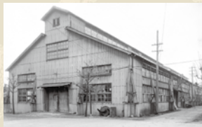
Former Toyo Seiki Head Office/Plant (Became ULVAC's Amagasaki Plant in 1956.)
