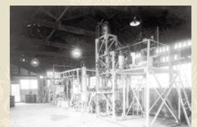
Product made by Toyo Seiki Molecular distillation equipment (Around 1948)
