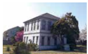
Still-standing Ward No. 1 of the Old Sanatorium (Part of the site is open to the public.)
