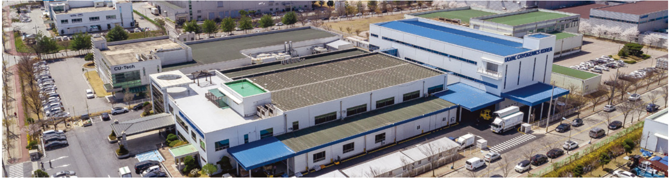
ULVAC CRYOGENICS KOREA INCORPORATED, exterior
