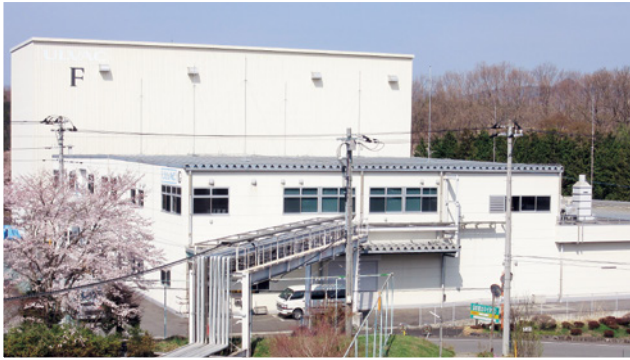
Exterior view of the FST site
