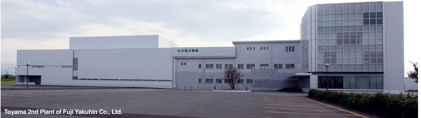
Toyama 2nd Plant of Fuji Yakuhin Co., Ltd.
