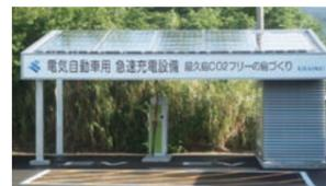
Electric vehicle quick-charging station with a power storage function
