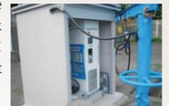
Quick-charging system for battery-powered boats
