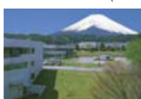
ULVAC Inc. Fuji Susono Plant/ Institute for Semiconductor & Electronics Technologies (Japan)
