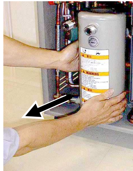
Figure 7-5 Connecting and disconnecting self-sealing coupling with two spanners
