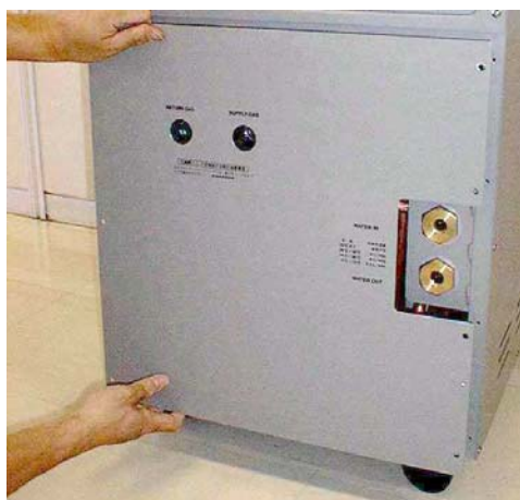
Figure 7-3 Remove the rear panel
