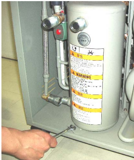
Figure 7-6 Remove adsorber mounting bolt
