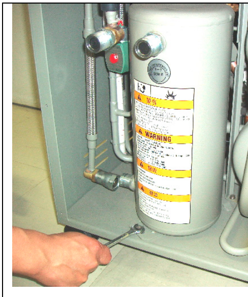
Figure 7-6 Remove the Bolt
