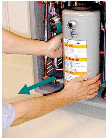
Figure 7-7 Slide out Adsorber Bottle
