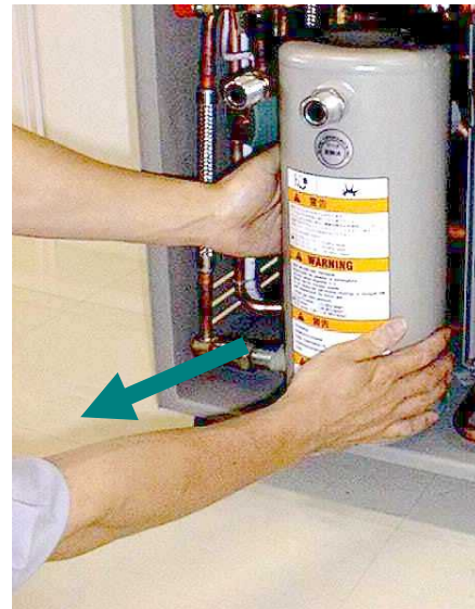
Figure 7-6 Remove adsorber mounting bolt (left)
