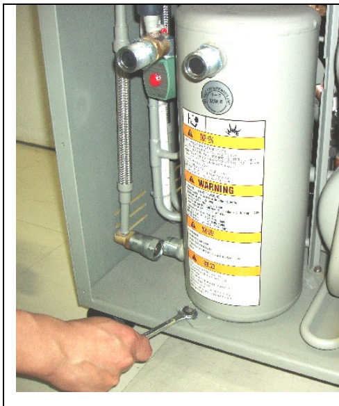
Figure 6-6 Remove the Bolt
