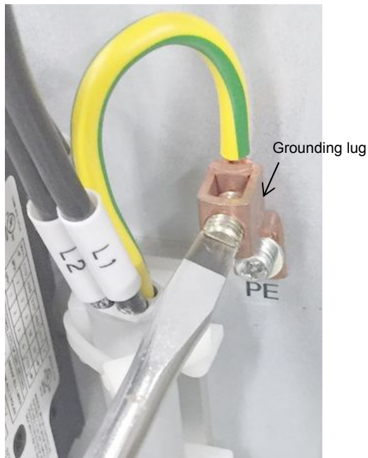
Figure 4-11 Connect Yellow and Green Earth Wires to Earth Terminal
