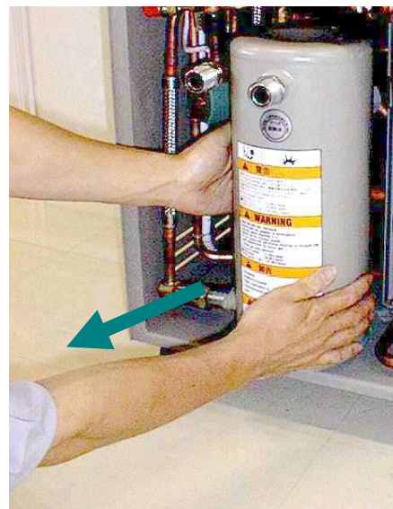
Figure 6-7 Slide out Adsorber Bottle
